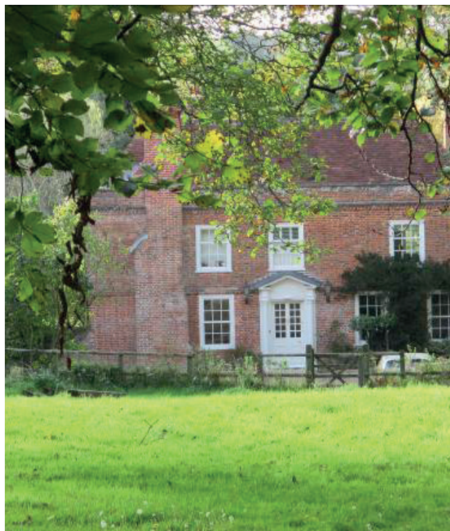
Church Farmhouse is typical of the attractive Georgian houses at the Northern end of the village.
