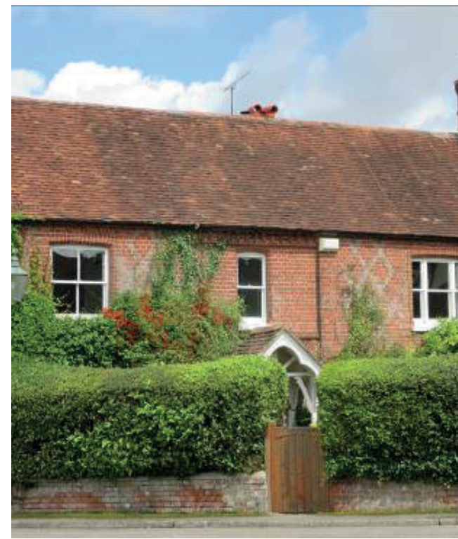
Enfield is a handsome house displaying various brickwork features including header bonding and diaper patterns.
