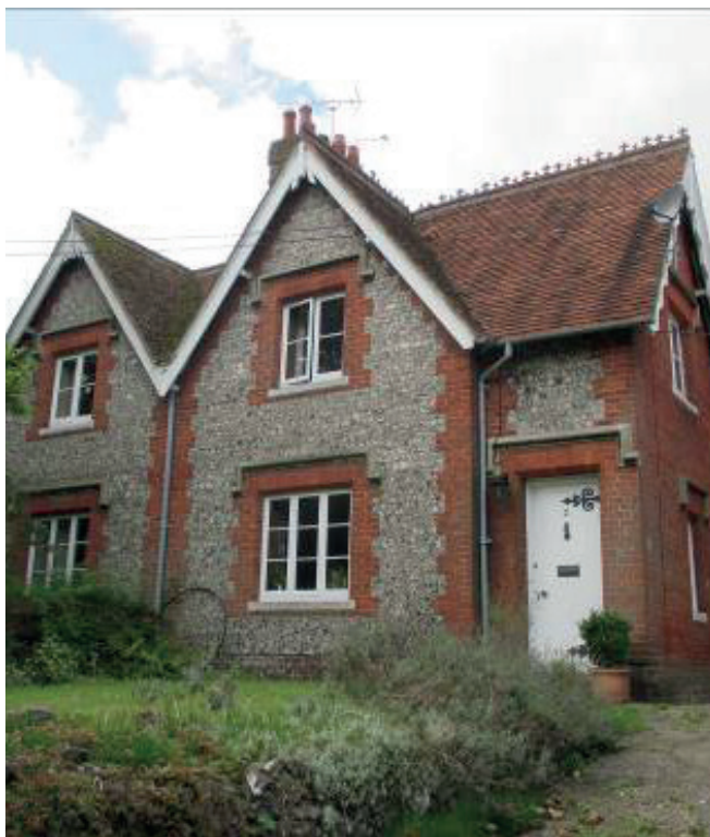
Beaulieu Cottages are a delightful pair of later Nineteenth Century properties making a strong positive contribution to the Conservation Area.
