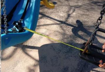
**Finding:** The seats are too close to each other as defined in **Action:** Monitor - No action given the risk assessment BS EN 1176 Part 2; this is a low risk failure and no remedial action is required
