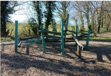
**Finding:** The timber edging forms a hard object within the falling space of the equipment and there is also insufficient surfacing provided in contravention of BS EN 1176 Part 1
