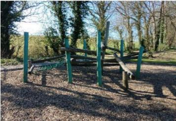
**Finding:** The depth of the loose fill surfacing is lower than the recommended depth specified in BS EN 1176; the free height of fall of the equipment is less than 2.0m and a minimum of 300mm depth should be provided (including an extra 100mm to allow for compaction and displacement as per BS EN 1176 Part 1 - Table 4)
