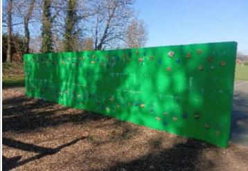
**Finding:** The safety surface is low and the membrane is exposed creating trip points
