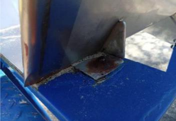
Finding: The fixings have corroded excessively
