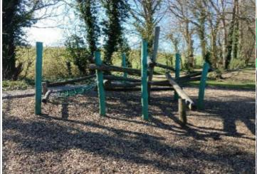
**Finding:** There are falls in excess of 600mm between adjacent components on the structure, in contravention of the recommendations set out in BS EN 1176 Part 1; 4.2.8.4
