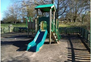
**Finding:** There is/are finger entrapment/s adjacent to the slide and the item fails to meet the requirements of BS EN 1176 Part 1 4.2.7.6 Entrapment of fingers
