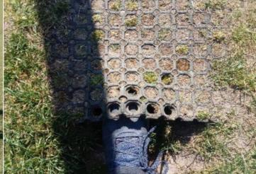
**Finding:** The surface is lifting at the edges and creating trip **Action:** Repair perimeter of surfacing to remove trip points points
