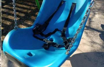
**Finding:** The safety harness is not designed to be left on the seat as it presents a strangulation risk if not used as intended. The manufacturer advises that the harness is an accessory that comes to the play area with the supervisor and leaves with the supervisor. The harness is not to be left attached to the seat when not in use.
