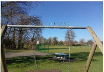
**Finding:** Swings of this design should have a secondary safety mechanism fitted to prevent collapse of the seat in the regularly event of a joint failure to comply with BS EN 1176 Part 2, however this swing was installed prior to the standards being updated in 2018 and the manufacturer has confirmed
