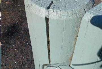
**Finding:** The timber has a number of splits/shakes or air cracks and this may affect the stability or allow water ingress fixing points of the structure and/or cause any instability which will accelerate the rotting process
